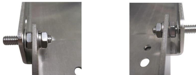
Hardware tightened in place
